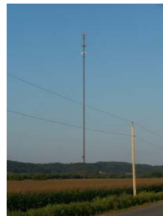
Cell Tower Located in the Town
